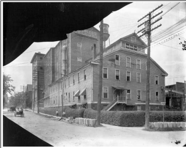
Figure 171: Peerless Flour Mill, no longer extant, photograph from Open Durham, accessed via http://www.opendurham.org/buildings/austin-heaton-flour-mill
