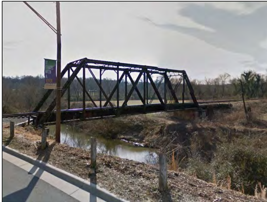
Figure 6: Big Elkin Creek Bridge, north elevation
