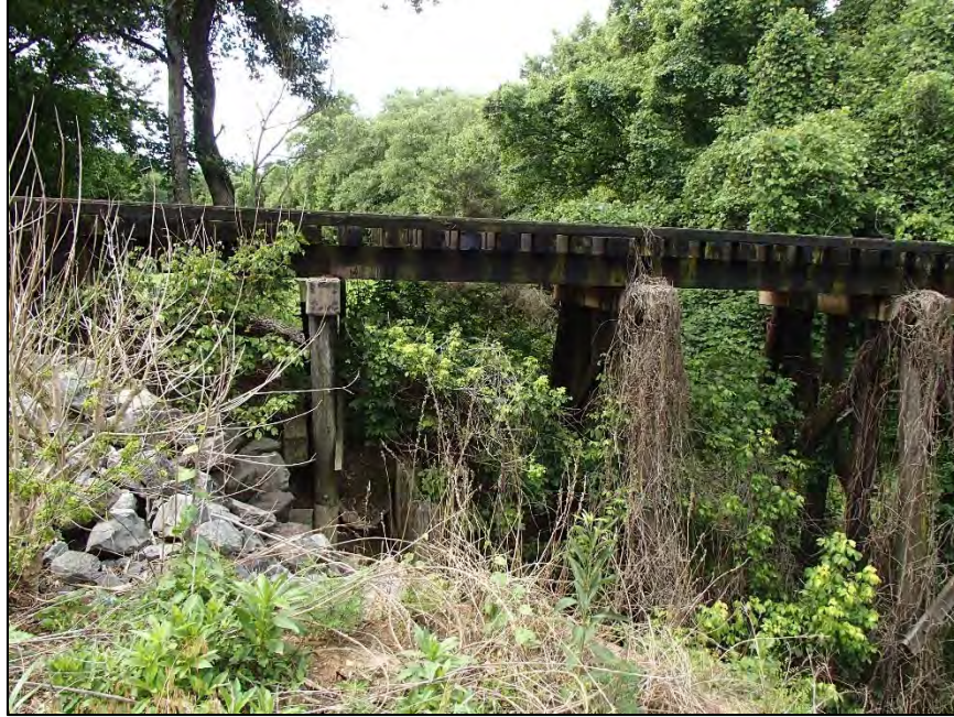
Figure 119: Bugaboo Creek Railroad Bridge, north elevation, east trestle section
