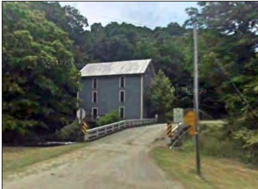
Figure 168: Helton Roller Mill, AH 59, 123 John Griffith Rd., Lansing vicinity, Google Streetview photo, June 2009
