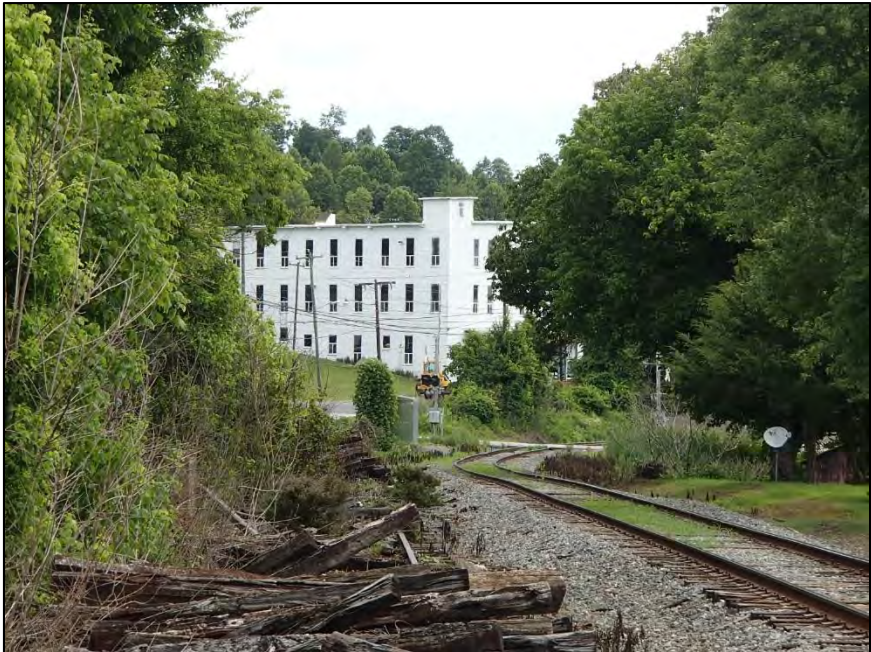
Figure 130: Ronda Historic District, Home Chair Company as seen from the railroad tracks at Main St
