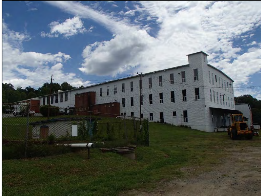
Figure 153: Home Chair Company, southwest corner
