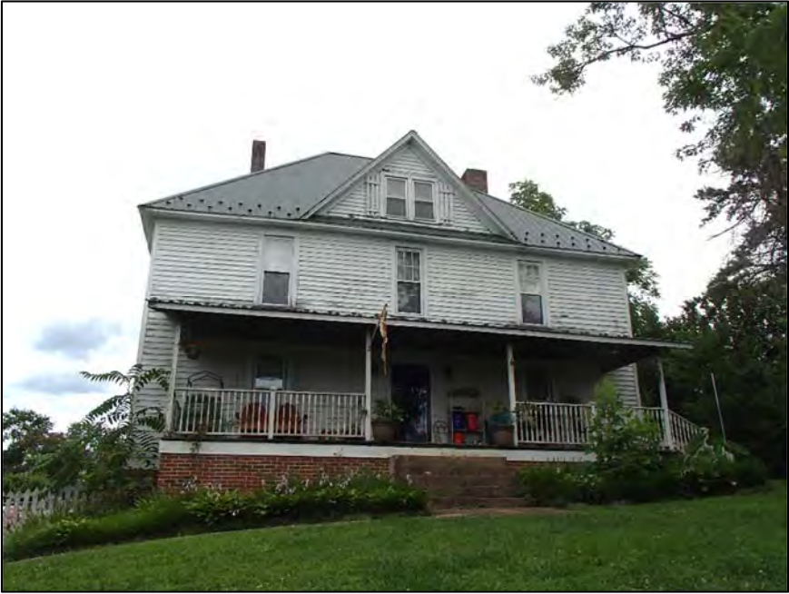
Figure 50: R.A. Reves House, south elevation
