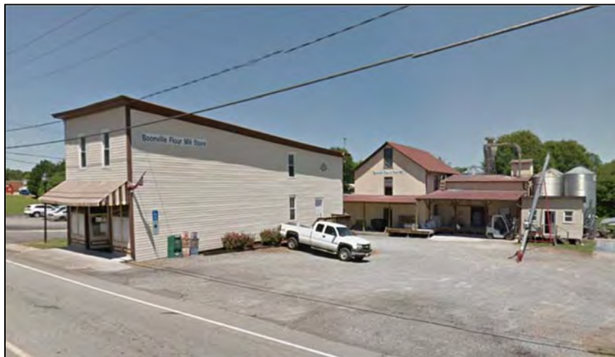
Figure 81: Booneville Feed Mill, YD 477), southeast corner of South Carolina Avenue and Academy Street, Google Streeview photograph, June 2016
