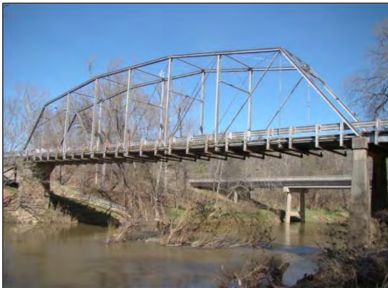
Figure 8: Deep River Camelback Bridge, photo by Matthew B. Ridpath, published at https://sites.google.com/site/matthewbridpath/bridges-and-highways-1/truss-bridges/deep-river-camelback-truss-bridge
