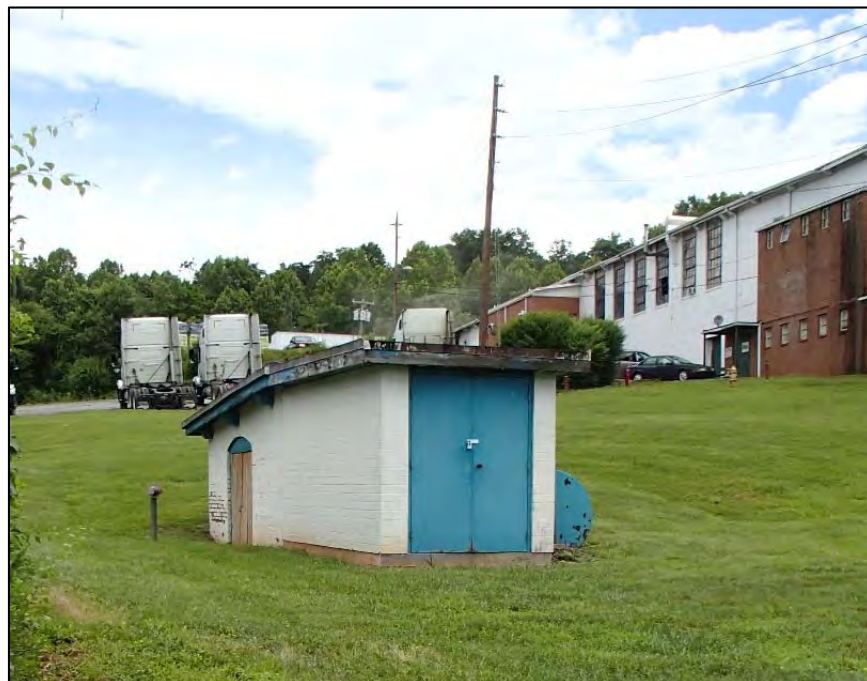
Figure 166: Home Chair Company, pump house
