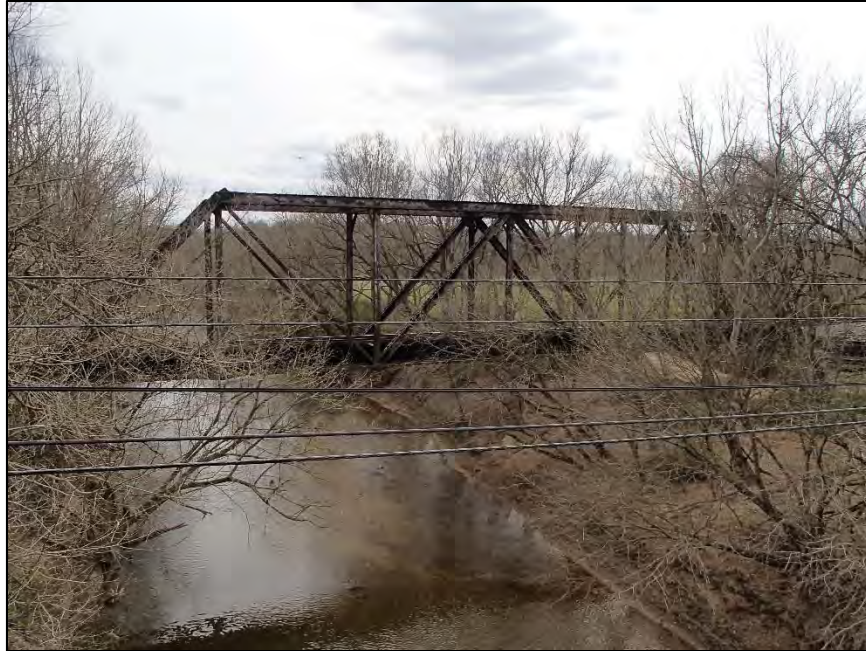
Figure 5: Roaring River Railroad Bridge, north elevation
