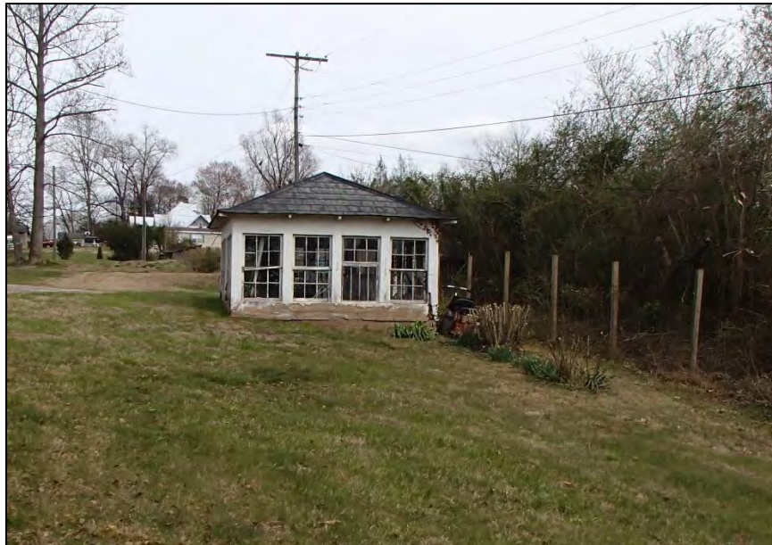
Figure 34: Reves-Greenwood Complex, J.E. and Matilda Greenwood House, flower pit
