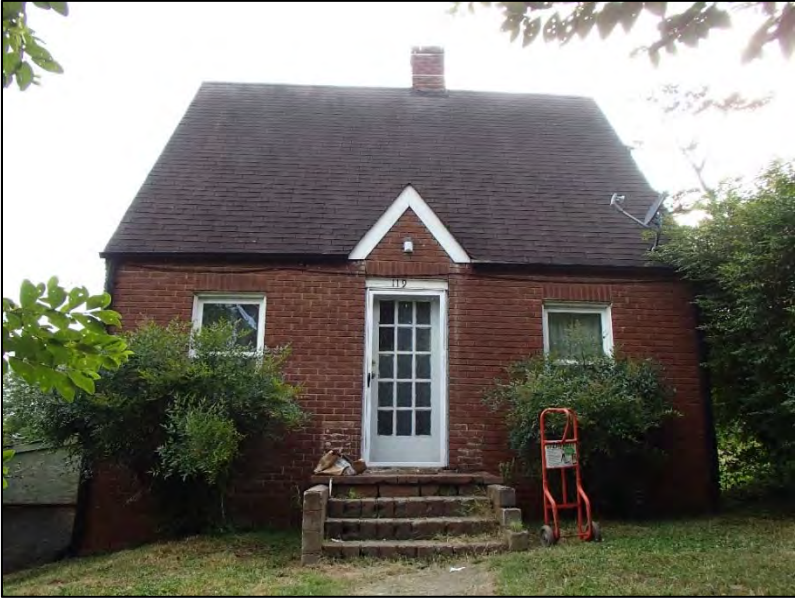
Figure 66: Roaring River United Methodist Church and Parsonage, house, east elevation
