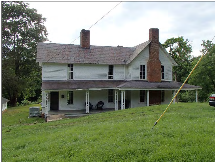
Figure 17: Reves-Greenwood Complex, Reves-Greenwood House, east elevation
