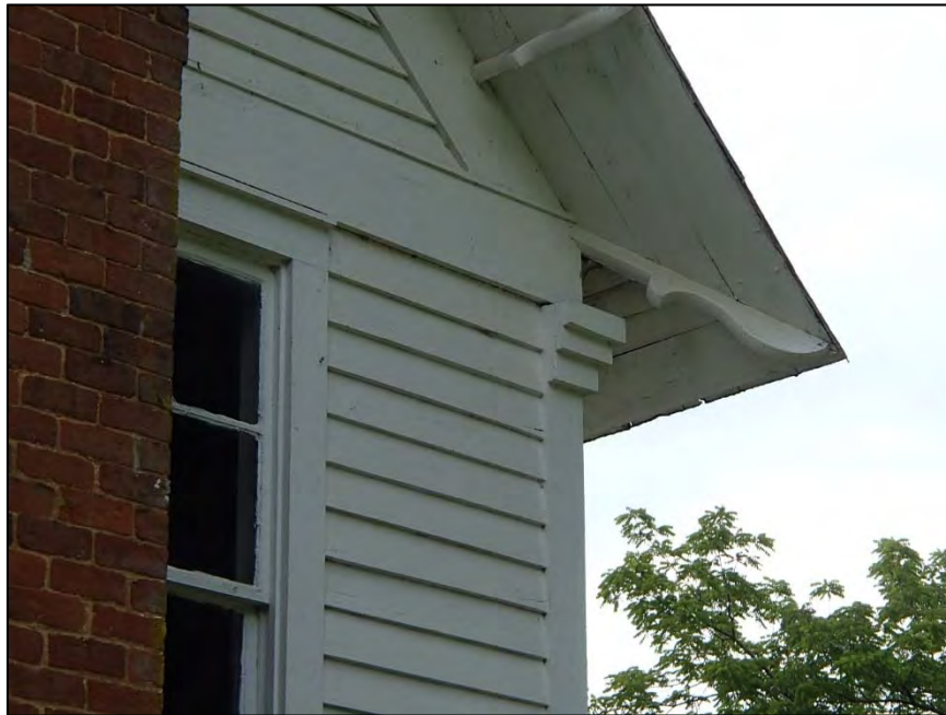
Figure 21: Reves-Greenwood Complex, Reves-Greenwood House, cornerboard and soffit detail
