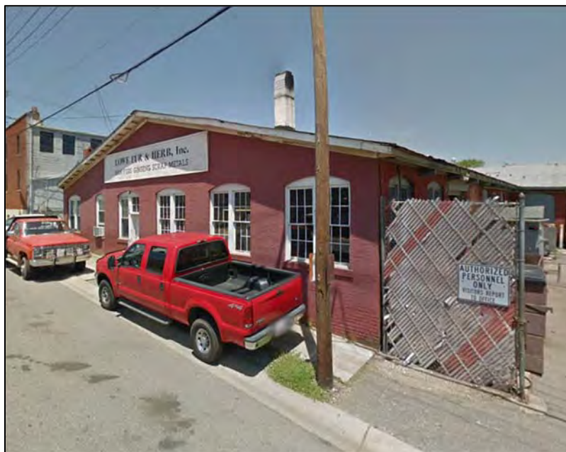
Figure 80: New Williams Mill, (WK 181), 108 Fifth Street, North Wilkesboro, Google Streetview photo, May 2013
