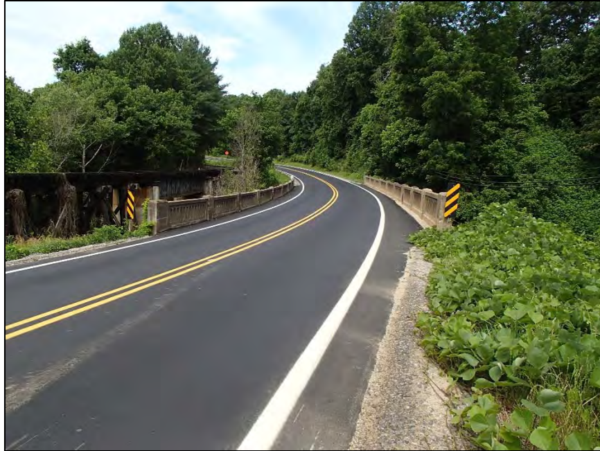
Figure 112: Bugaboo Creek Bridge, facing west
