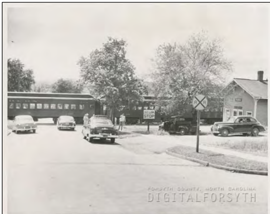
Figure 137: 1955 photo of last passenger train stop in Ronda, showing depot, Frank Jones photographer, from the photo collection at the Forsyth County Public library, accessed via Digital Forsyth, http://www.digitalforsyth.org/photos/2889
