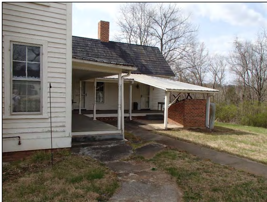
Figure 33: Reves-Greenwood Complex, J.E. and Matilda Greenwood House, rear ell
