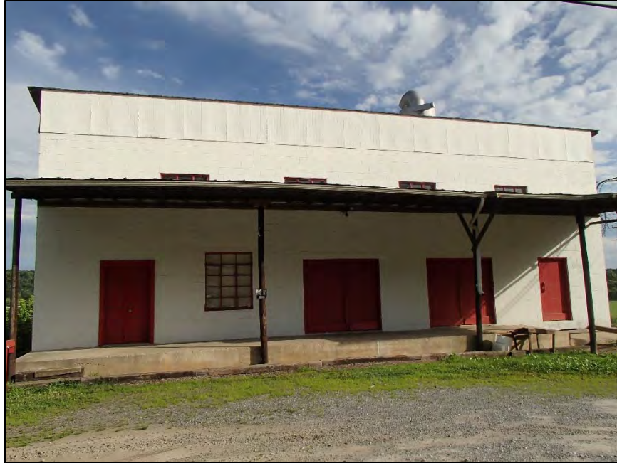
Figure 74: Roaring River Milling Company, north elevation
