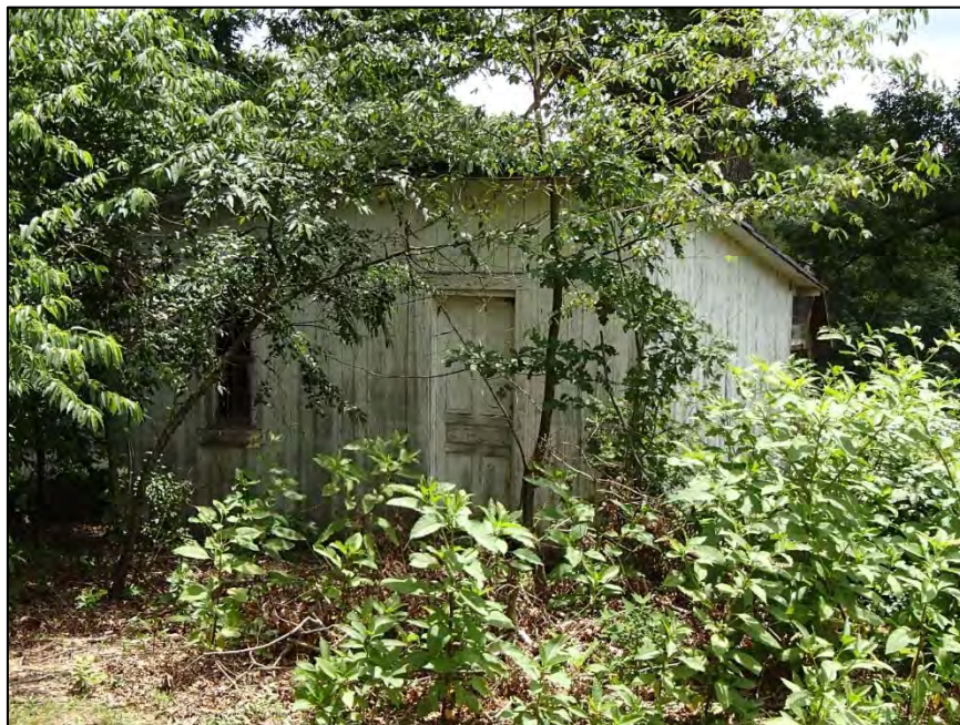
Figure 183: Poplin Family Farm, cottage shed
