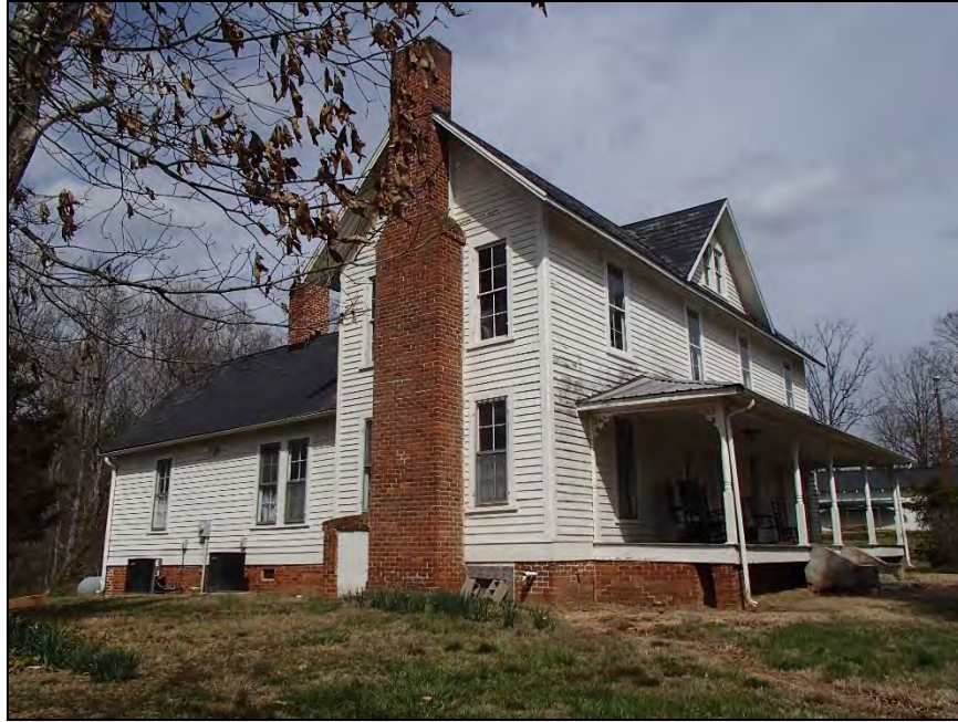
Figure 31: Reves-Greenwood Complex, J.E. and Matilda Greenwood House, southwest corner
