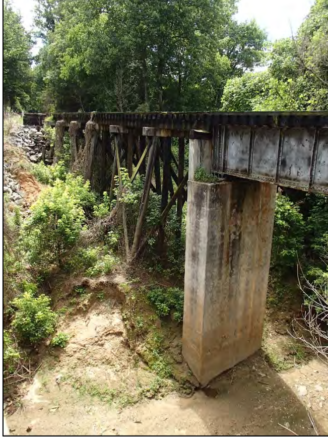
Figure 121: Bugaboo Creek Railroad Bridge, facing southeast
