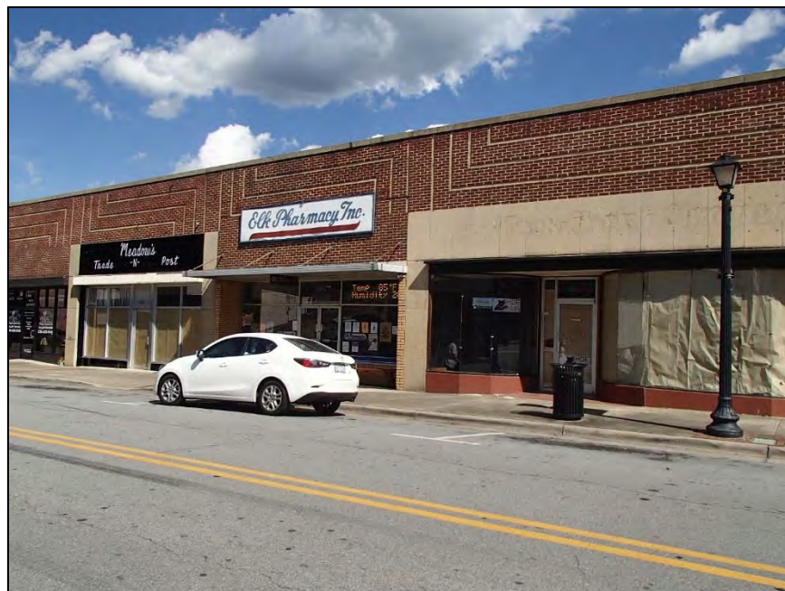
Figure 204: 100 block of East Main Street,, SR 823, Elkin
