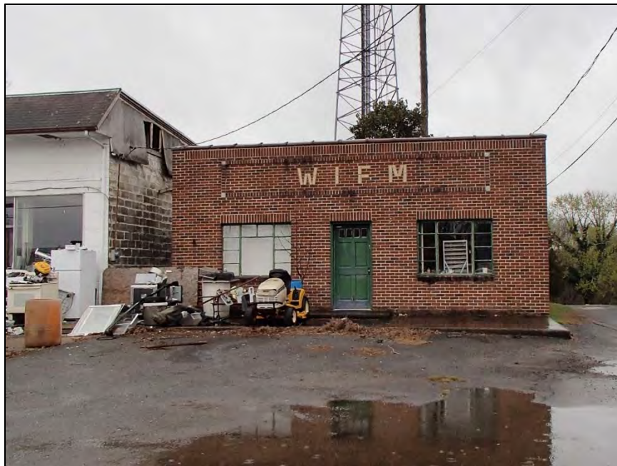
Figure 200: WIFM Radio Station, north elevation
