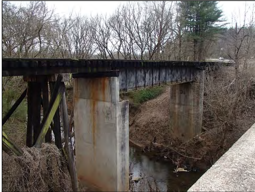
Figure 120: Bugaboo Creek Railroad Bridge, north elevation, girder bridge
