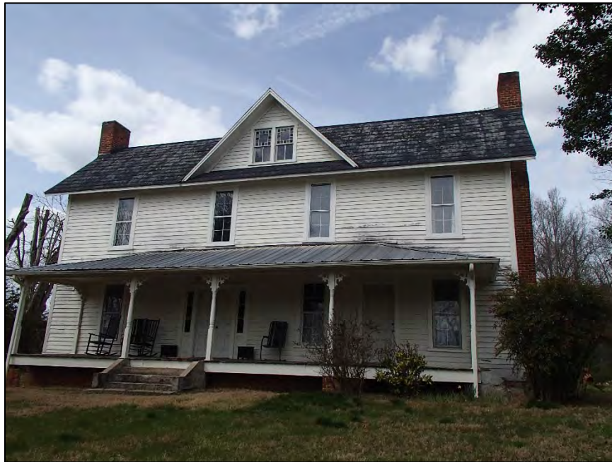
Figure 30: Reves-Greenwood Complex, J.E. and Matilda Greenwood House, south elevation
