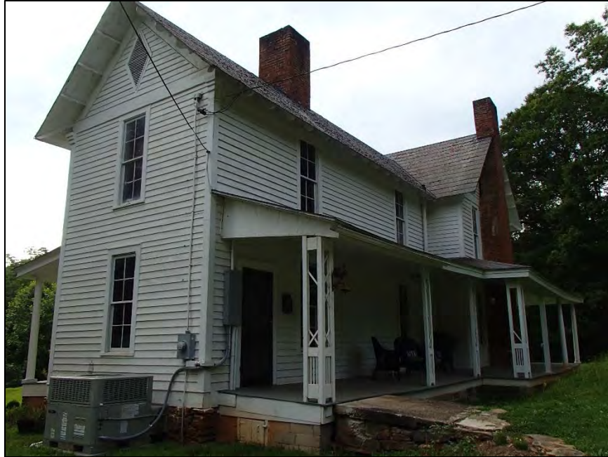
Figure 19: Reves-Greenwood Complex, Reves-Greenwood House, southeast corner
