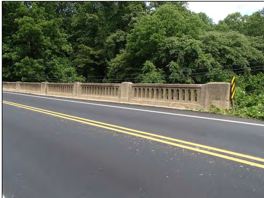
Figure 113: Bugaboo Creek Bridge, north railing
