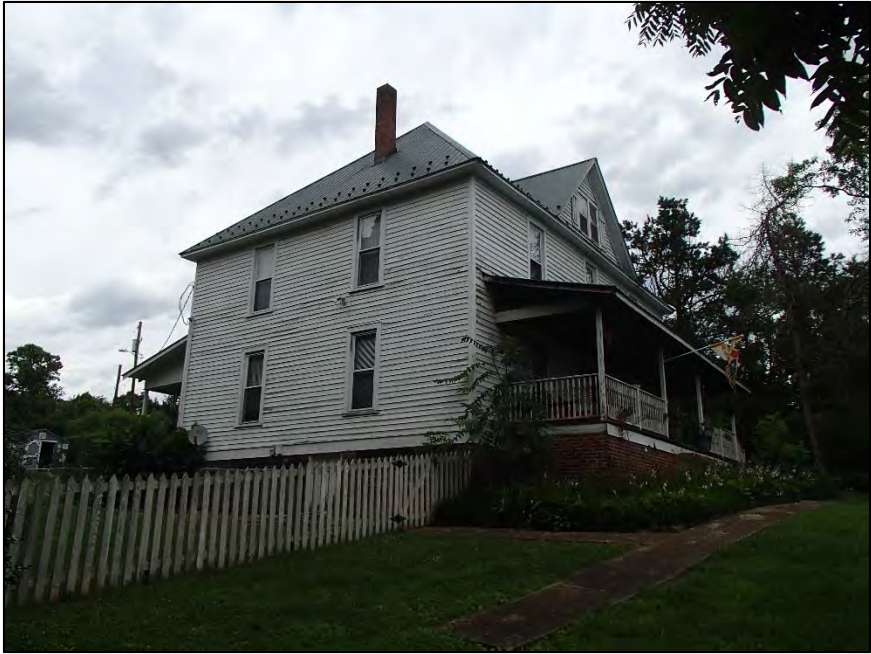
Figure 51: R.A. Reves House, southwest corner
