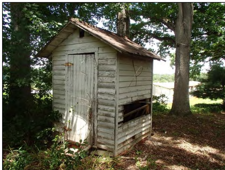
Figure 181: Poplin Family Farm, carbide generator house
