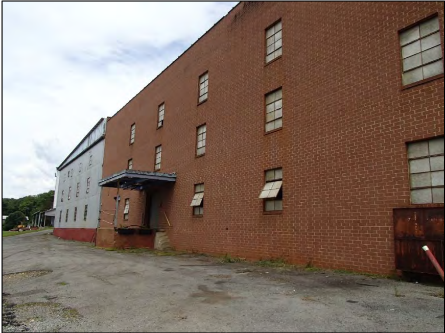
Figure 162: Home Chair Company, 1940s section with ca. 1950 addition, south elevation
