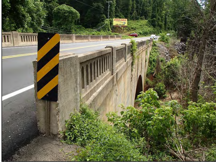
Figure 114: Bugaboo Creek Bridge, south elevation
