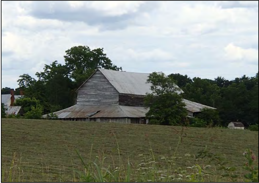
Figure 44: Farm, 2226 Tharpe Rd.
