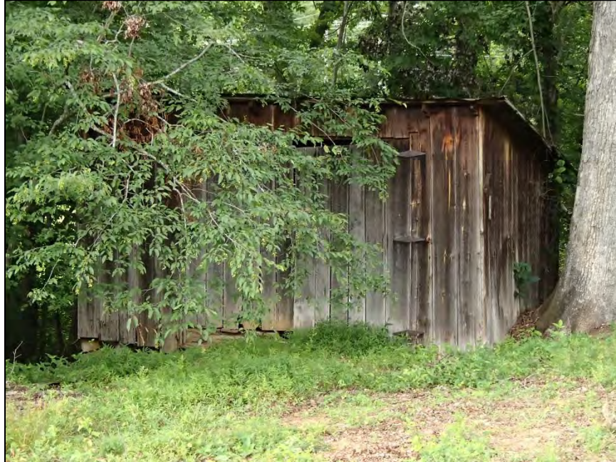
Figure 28: Reves-Greenwood Complex, Reves-Greenwood House, shed
