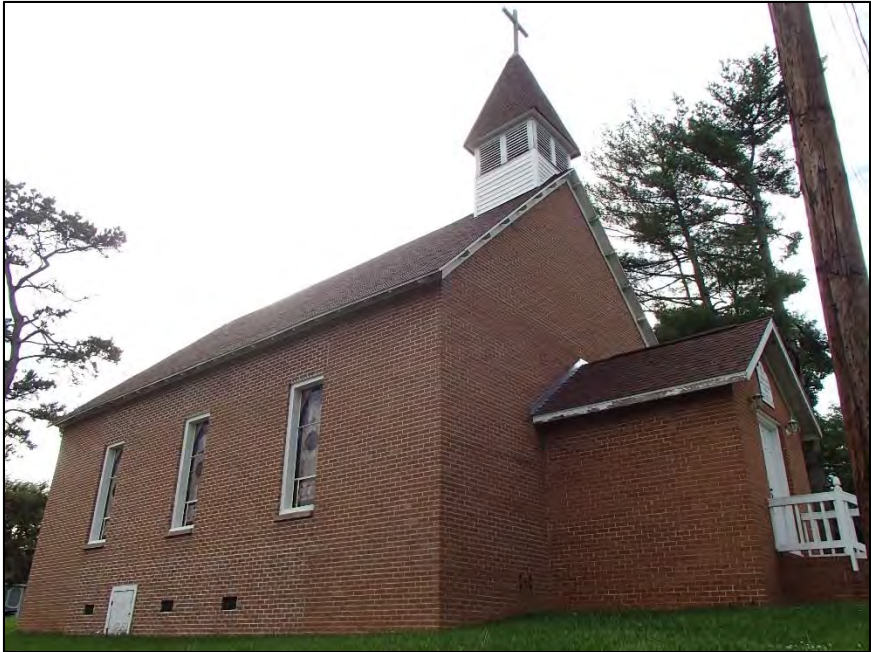
Figure 61: Roaring River United Methodist Church and Parsonage, southeast corner
