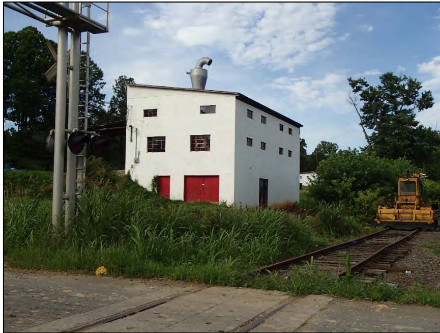
Figure 76: Roaring River Milling Company, southwest corner
