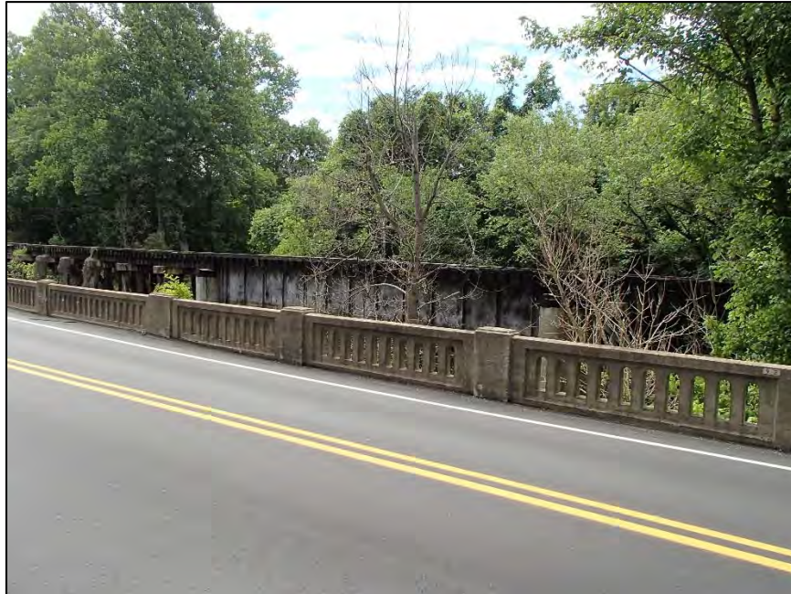
Figure 115: Bugaboo Creek Bridge, south railing
