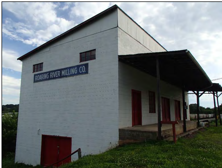
Figure 75: Roaring River Milling Company, east elevation
