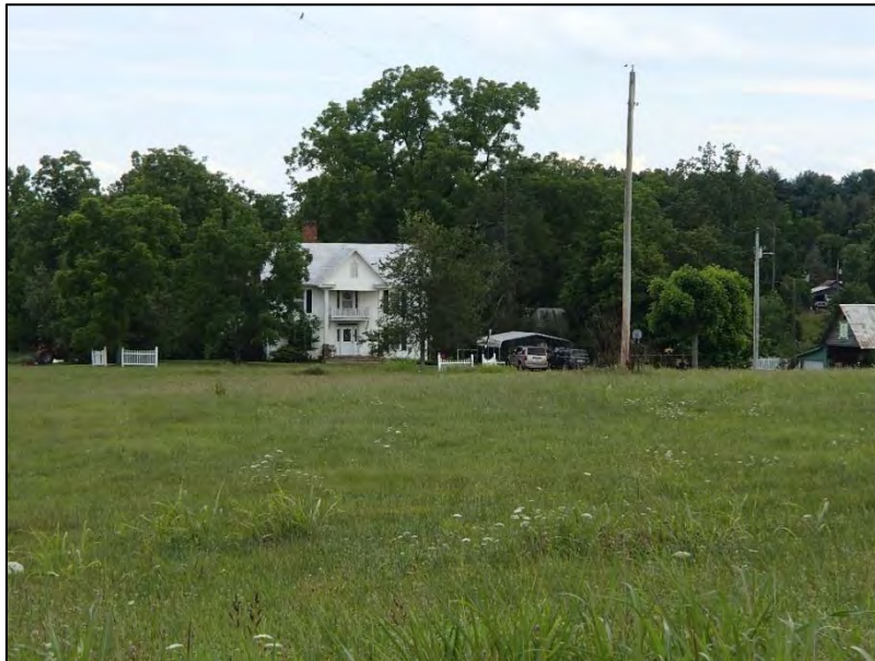
Figure 105: Farm at 2226 Tharpe Rd.
