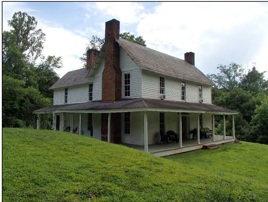
Figure 16: Reves-Greenwood Complex, Reves-Greenwood House, northeast corner
