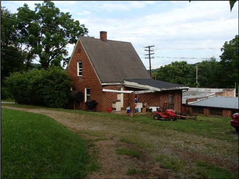
Figure 67: Roaring River United Methodist Church and Parsonage, house, northwest corner
