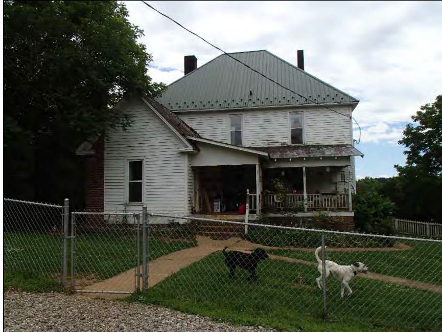
Figure 53: R.A. Reves House, north elevation
