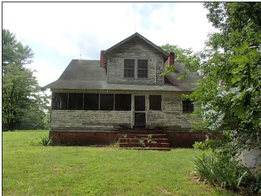
Figure 179: Poplin Family Farm, main house, east elevation
