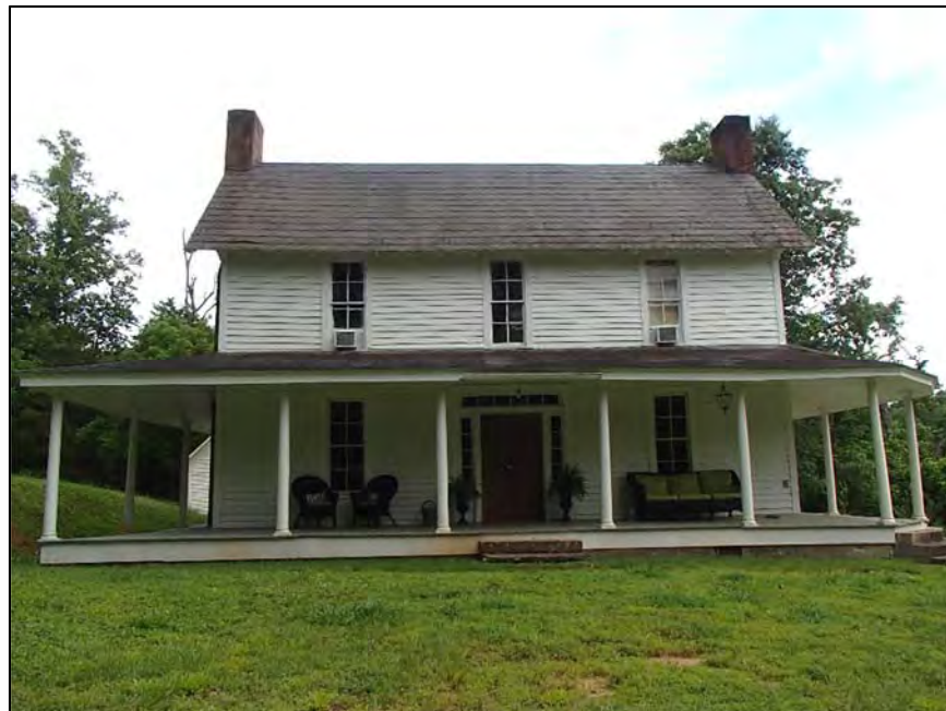
Figure 14: Reves-Greenwood Complex, Reves-Greenwood House, north elevation
