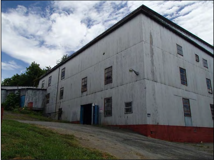
Figure 161: Home Chair Company, ca. 1940 building, southwest corner
