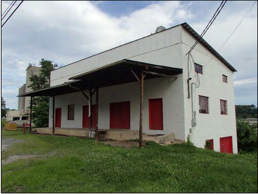
Figure 72: Roaring River Milling Company, northwest corner
