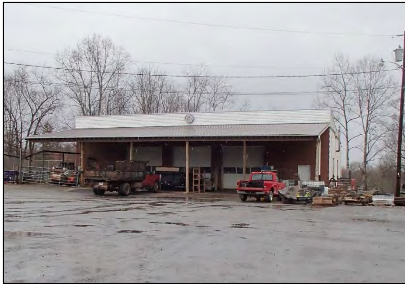
Figure 79: Possible feed mill building at the Farm Supply Store, 15846 Elkin Highway
