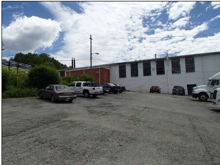
Figure 158: Home Chair Company, 1940s junction between original section and the ca. 1960 addition, west elevation
