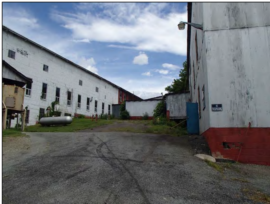
Figure 164: Home Chair Company, original section to the left; ca. 1940 building to right
