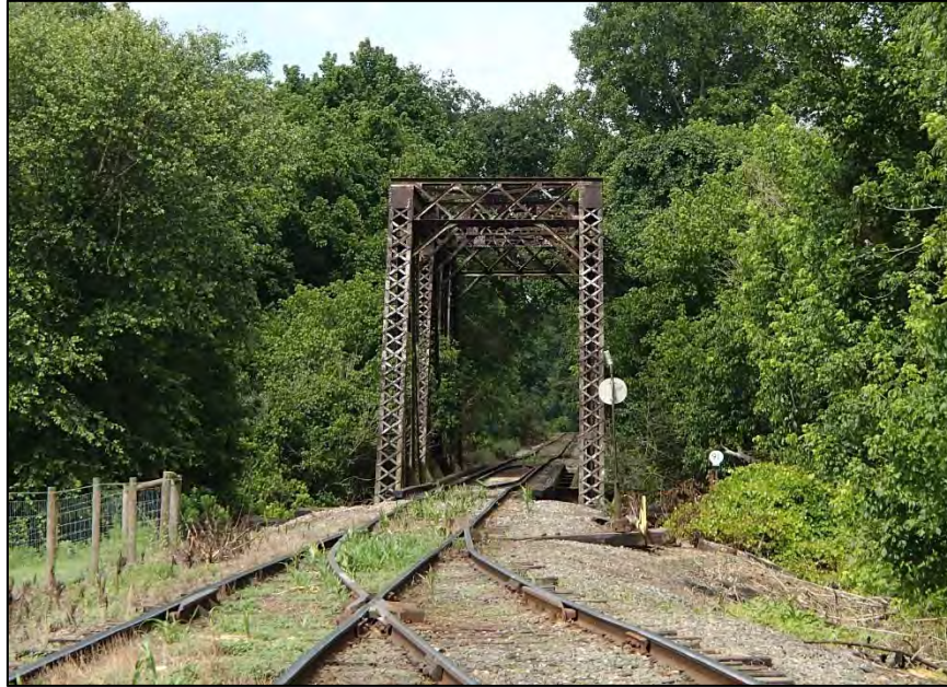
Figure 4: Roaring River Railroad Bridge, east elevation
