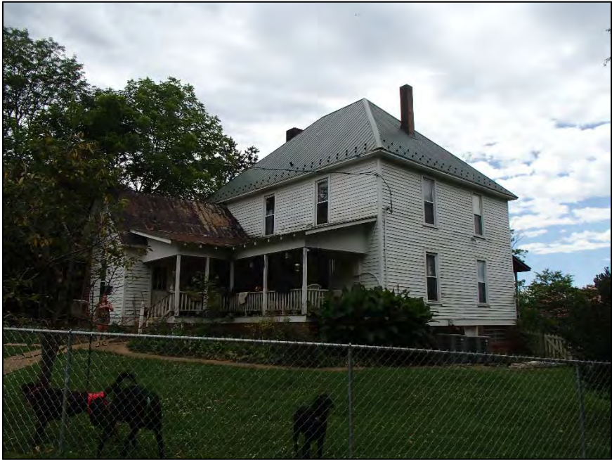
Figure 52: R.A. Reves House, northwest corner
