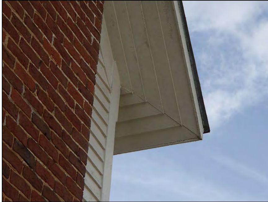
Figure 32: Reves-Greenwood Complex, J.E. and Matilda Greenwood House, soffit detail
