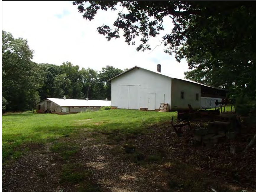
Figure 184: Poplin Family Farm, south chicken houses; 1948 house is closer, 1960s house in distance
