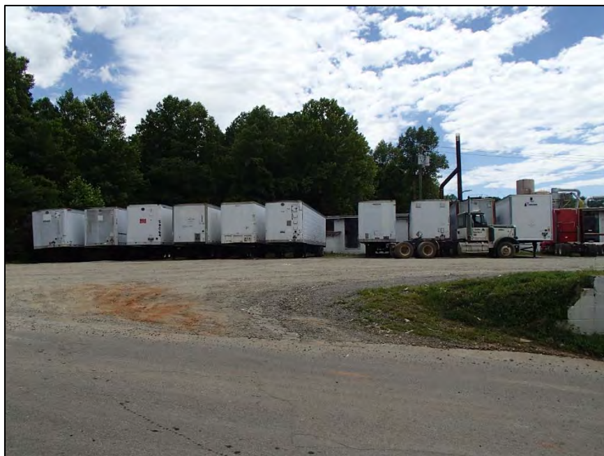
Figure 160: Home Chair Company, ca. 1960 section, west elevation behind trucks
