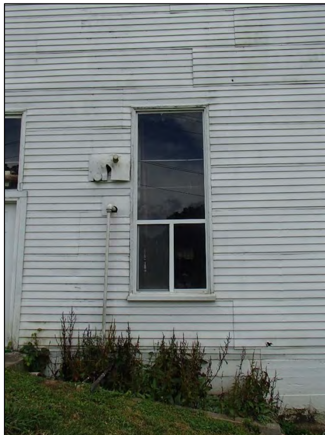
Figure 154: Home Chair Company, replacement window detail
