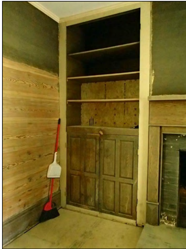
Figure 22: Reves-Greenwood Complex, Reves-Greenwood House, built-in cabinet
