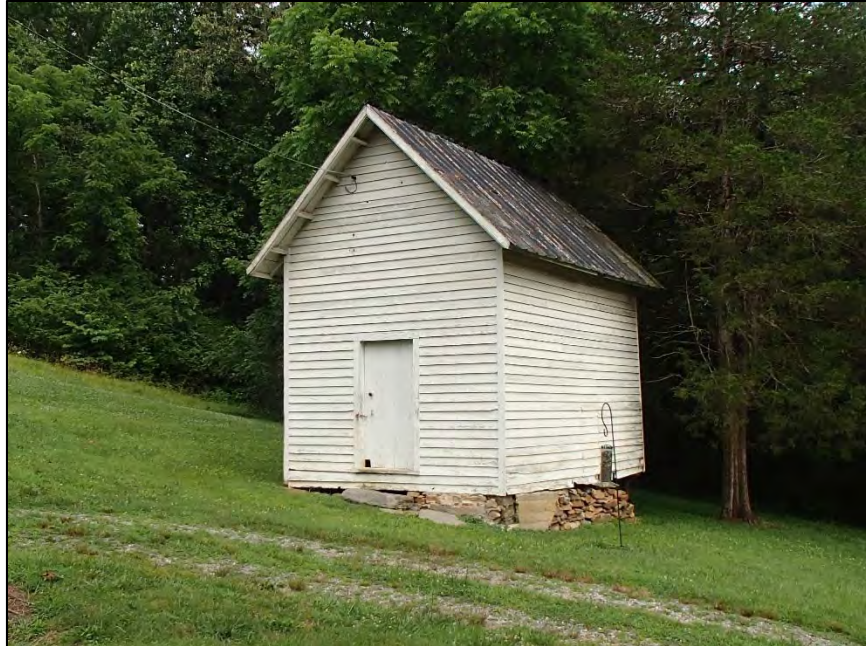
Figure 26: Reves-Greenwood Complex, Reves-Greenwood House, outbuilding
