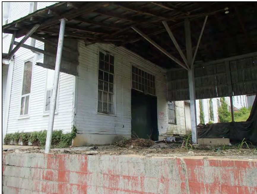
Figure 156: Home Chair Company, southeast corner with original windows and doors
