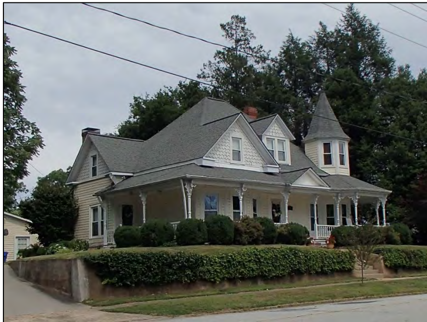
Figure 40: Caudill House, WK 74, 710 9th Street, North Wilkesboro
