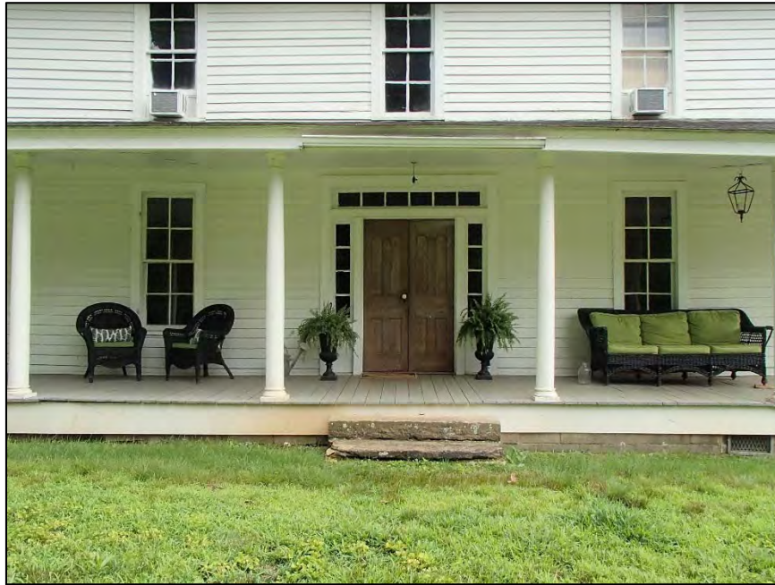
Figure 15: Reves-Greenwood Complex, Reves-Greenwood House, north elevation detail
