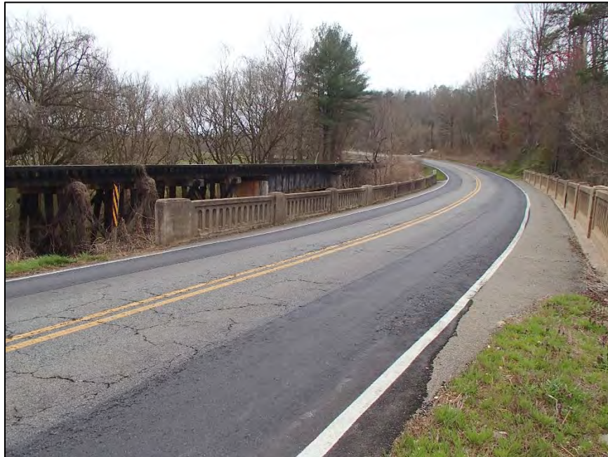
Figure 122: Bugaboo Creek Railroad Bridge, as seen from the highway bridge
