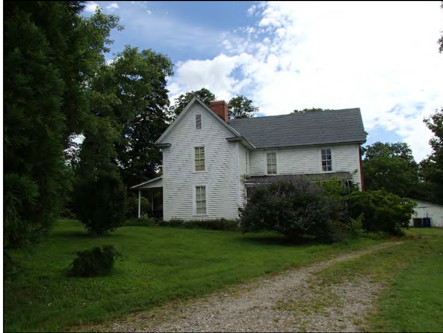
Figure 144: Ronda Historic District, 221 Main St.
