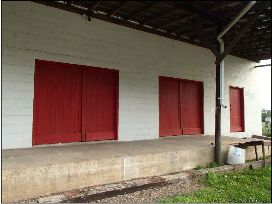
Figure 73: Roaring River Milling Company, north elevation detail
