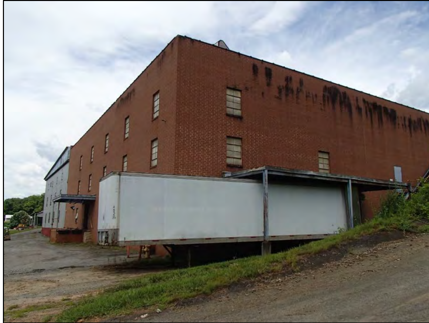
Figure 163: Home Chair Company, ca. 1950 addition, southeast corner
